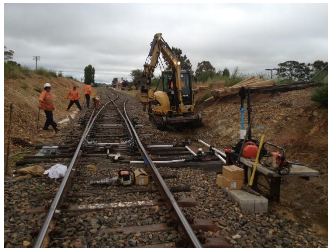
Turnout Maintenance Bungendore
