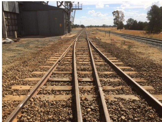
Turnout timbers put in at Aria Park
